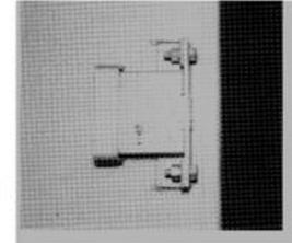
Fastenings must be appropriate to the size and structure. 'Rawl' and expanding bolts should be utilised in stone, brick and concrete. Coach screws and bolts for timber joists. The cabinet manufacturers will usually include recommendations for fixing devices
