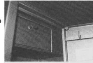
Any internal compartments for the storing of ammunition rifle bolts, etc. should be as strong as the main body of the cabinet
