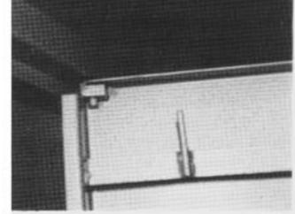
Cabinets with exposed hinge barrels and those with piano hinges which have been fitted using rivets require anti-prise plates.
